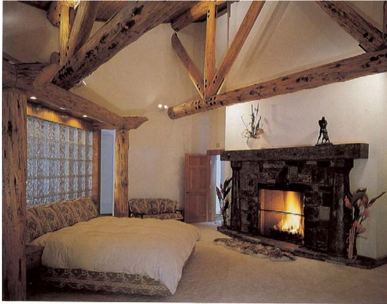
Below: See-through fireplace with birch log mantles serves dining room and sitting room, opposite side. Glue-laminated log beams on ceiling are original square beams reinforced on each side with steel and disguised in a round shape with cedar bark.
